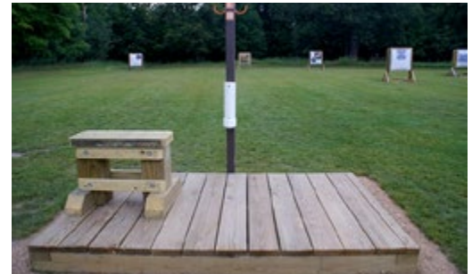
↑ Raised platform. Carver Park Reserve, Victoria, Minn.
